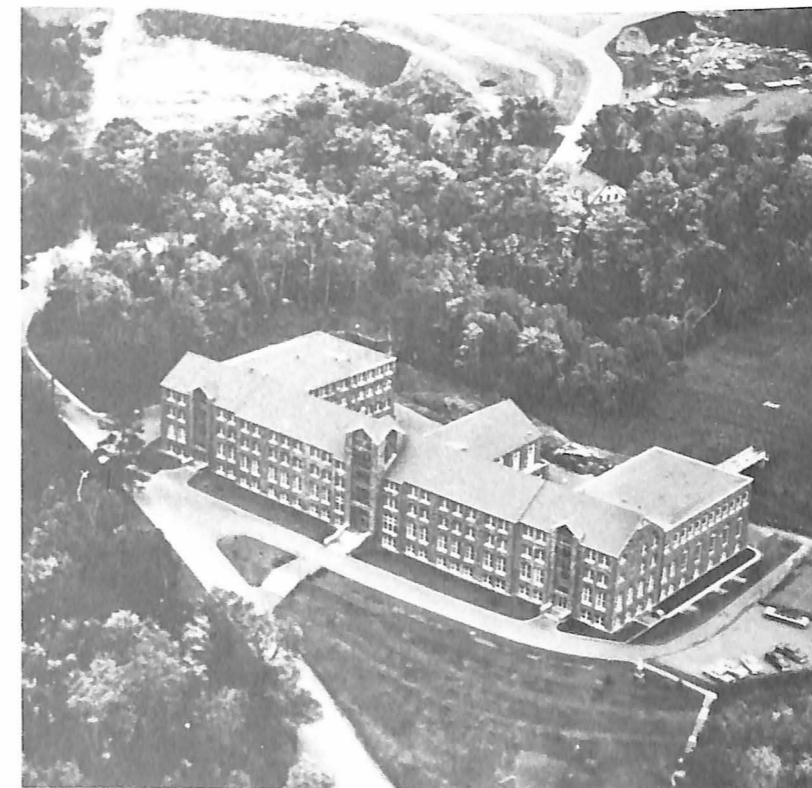
The new Evaristus after the fire.
