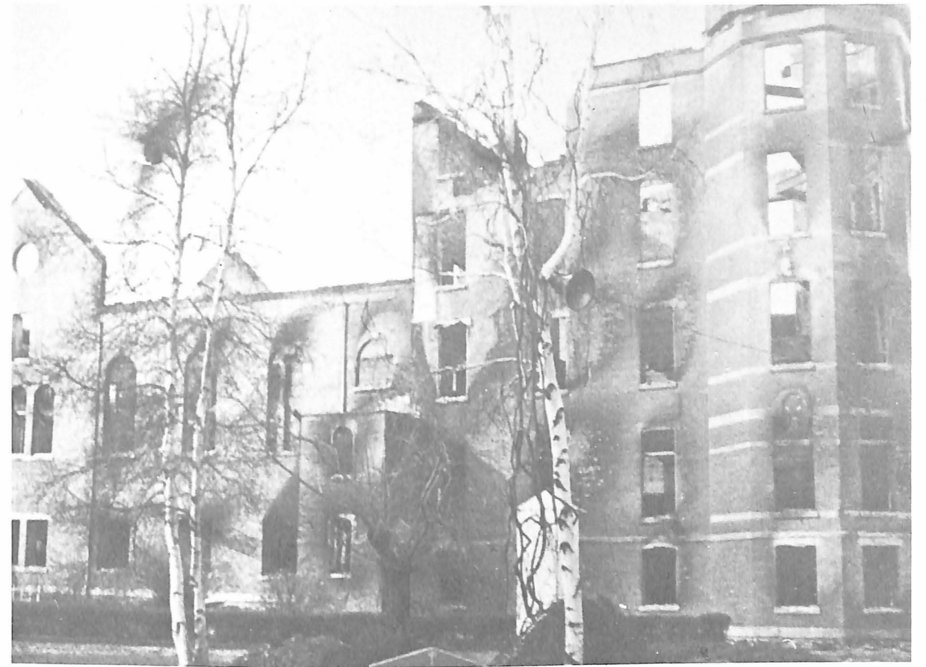
Fire completely destroyed this Mount building on a historic night in January 1951.
